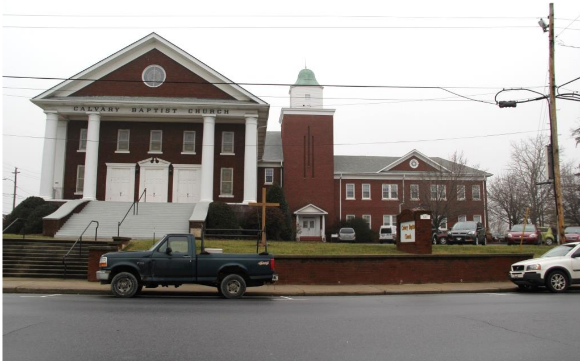
Calvary Baptist Church (BN4921), 531 Haywood Road, view to north. Photo by author, 2015.
